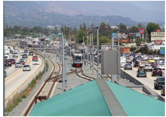
Figure 1 I-210 Freeway and Metro Light Rail in Los Angeles County
