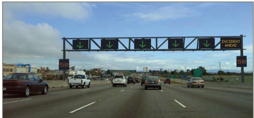
Project visual simulation with proposed sign bridge structure (gantry)
