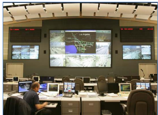
Figure 27 – Los Angeles Regional Transportation Management Center
