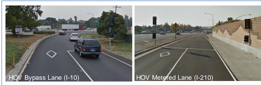
Figure 42 – Examples of HOV Bypass and HOV Metered Lanes on Freeway Ramps
