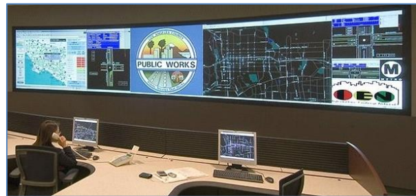
Figure 28 – Los Angeles County Traffic Management Center
