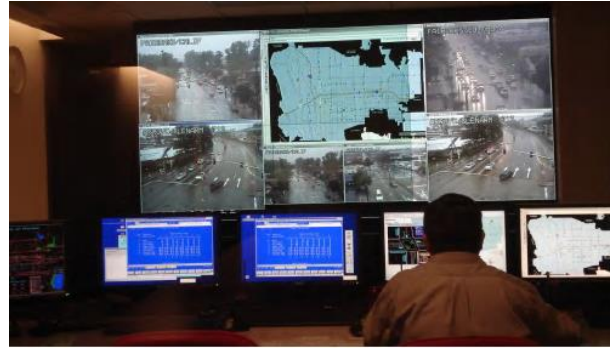
Figure 29 – Pasadena Traffic Management Center
