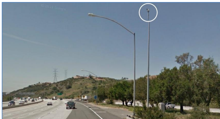
Figure 37 – CCTV Camera along I-210 West at SR-57 Interchange
